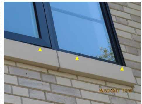
Front; drip flashing at bottom installed too short; should extend past the lower window trim for effective drainage.
