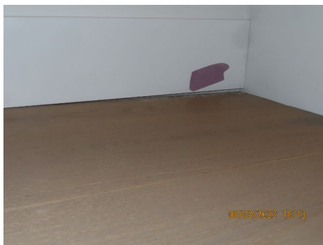
2nd floor closet - poor trim work finishing
