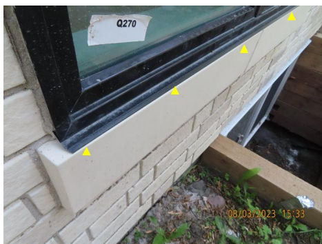
Front; recommend repair; drip edge too short; should extend past window trim for proper drainage.
