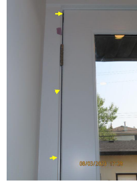
Rear exterior door to deck; recommend review for better fitting/ larger gap at top of door compared to lower.
