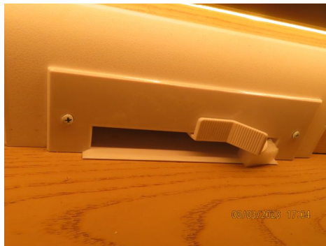
Floor sweep; not functional - no Cental VAC installed
