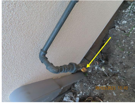
Additional gas line fitted for future gas space heater.
