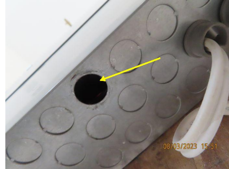
Missing panel plug; recommend installation for safety
