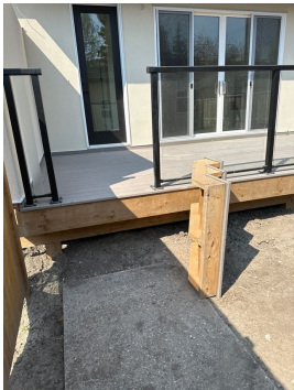
Rear deck stairs not installed at time of inspection.
