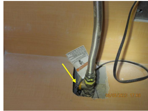
Difficult to rear the gas shutoff! Recommend repairs for safety.
