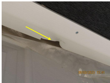
Damaged weatherstripping recommend replacement
