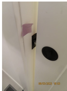
Door does not latch, needs adjustment. Location: 2nd floor bath/pocket door
