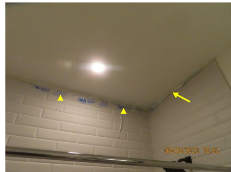
2nd floor main bath - remove tape at top; seal top of tilework
