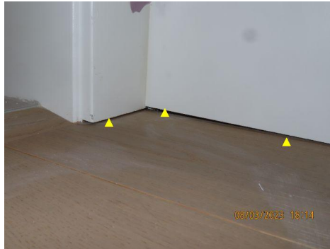
2nd floor closet; poor trim work
