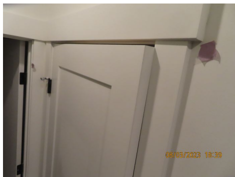
Basement; furnace room; not closing properly. Missing screws in hinge not installed. Repair advised.
