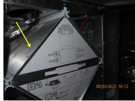
HRV - Missing one filter/ not installed - recommend installation
