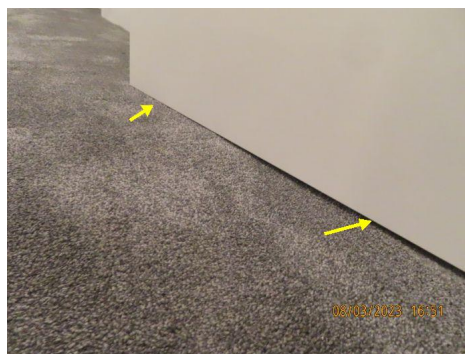
Basement bedroom - poor installation; door rubs against carpeting
