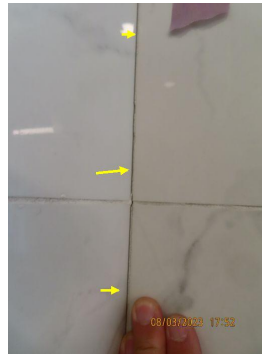
2nd floor ensuite bath: Missing grout/silicon glue seal
