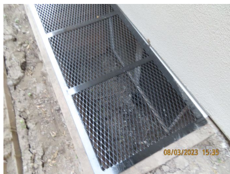
Exterior window covers are not secure and move; recommend review by builder to ensure safety.
