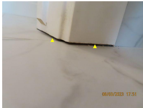
2nd floor bathroom - short trim work at door
