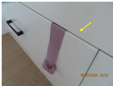
Master bedroom - window drawer - not closing flush
