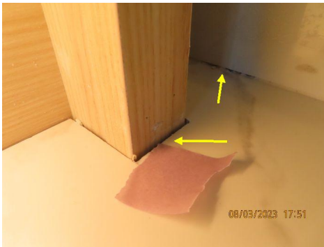
2nd floor bathroom - gaps around cabinetry; should be sealed to prevent moisture penetration into sub-flooring
