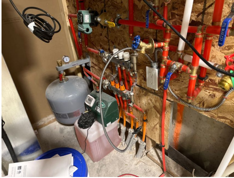
Multi Zone In-Floor Radiant Heating plumbing present in basement. Condition: NO seperated water tank to supply in floor radiant hearing. *Recommend reviewing current setup with builder as this system is not completed.
