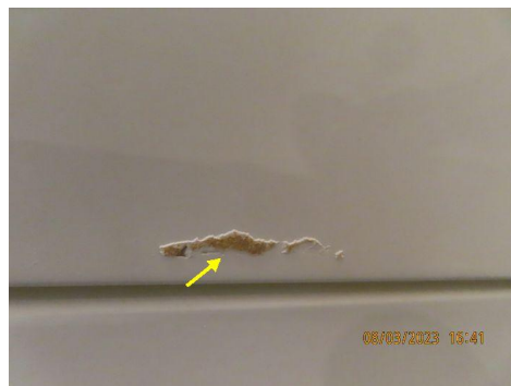
Damaged surface at basement built in - recommend repairs
